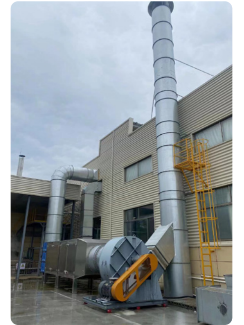
Upgrade of the decorative exhaust pipe de-dusting equipment
